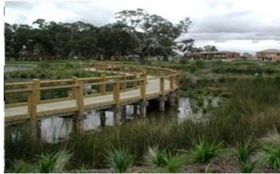
Lynbrook Estate stormwater wetland, Melbourne
