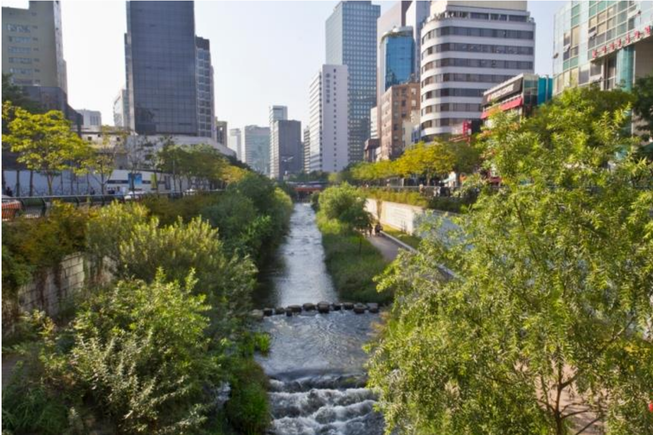
Cheonggyecheon stream in Seoul, South Korea, daylighted from sewers in 2003. Image: Kaizer Rangwala, Flickr.
